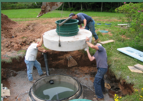
Pump station installation.
