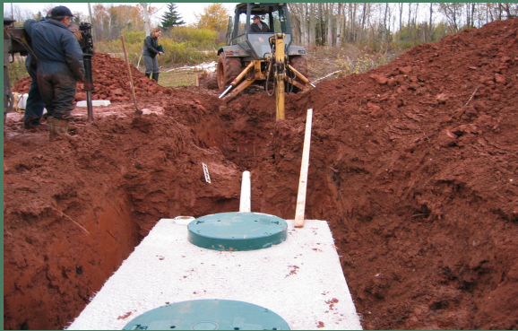
Septic tank and pump tank installation.
