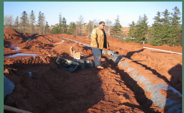
Leaching chambers installed in approved fill.
